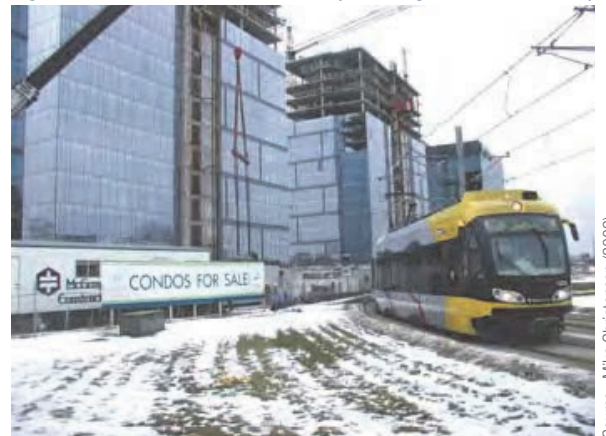
Figure 6. Reflections Condominiums (Bloomington Central Station)
